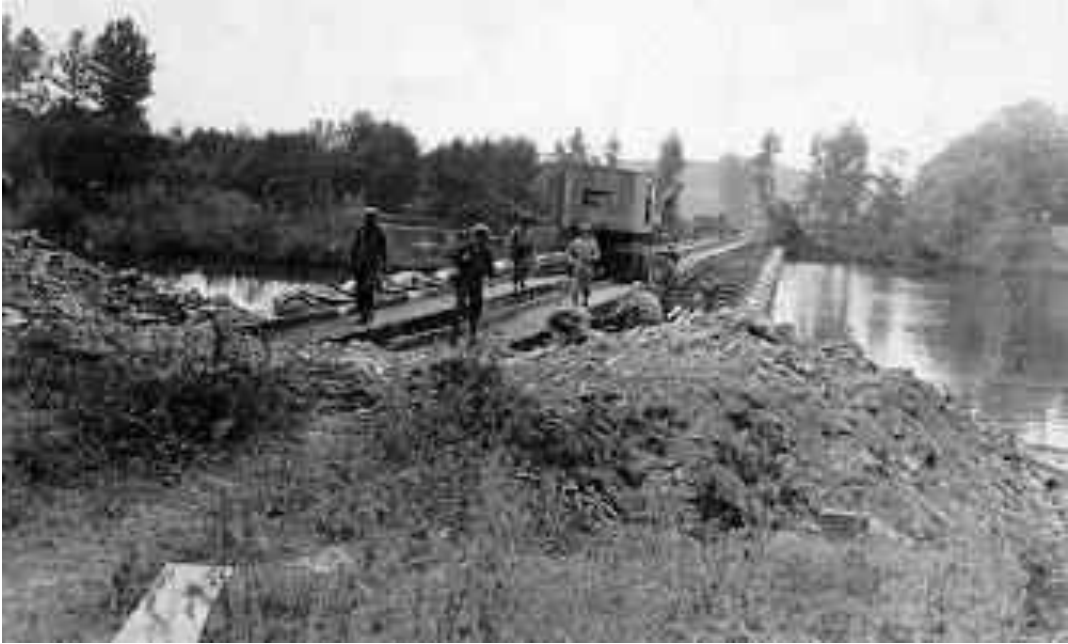
Photos of the Bridge over the Moselle River near Dieuouard, France.
